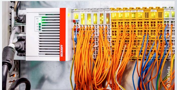
The control core of the PTL 4001 fiber laser cutting system comprises a CX5130 Embedded PC with TwinCAT 3 software and a wide range of EtherCAT Terminals, such as EL1904 TwinSAFE Terminals and EL3161 analog input terminals.
