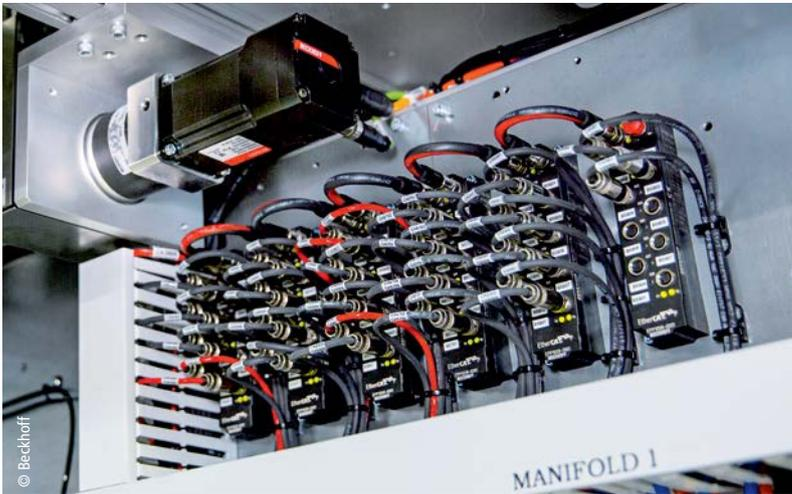
Left: IP67-rated EtherCAT Box modules use One Cable Automation via EtherCAT P to provide power and communication in a single cable.
