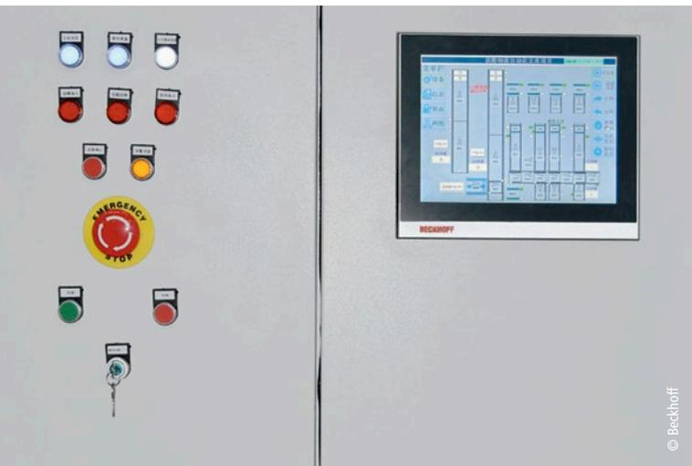
The Embedded PC in the control cabinet is connected to a Beckhoff Control Panel CP2912 used as HMI.
